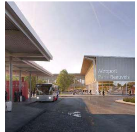
Paris Beauvais International Airport - France (completion expected 2029) • 24,000m 2 terminal extension • 2,000 new car parking spaces • 6 new aircraft stands
